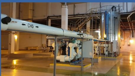
The Phase-Change Material thermal energy storage system co-developed by NUS has been installed at Keppel DHCS' Changi Business Park District Cooling System Plant.
